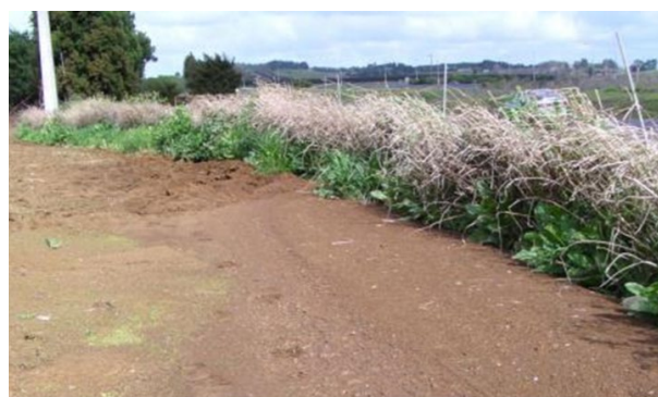
Figure 3.7: Example of vetiver grass being used as a soil barrier (photo credit - Master & Sons).
