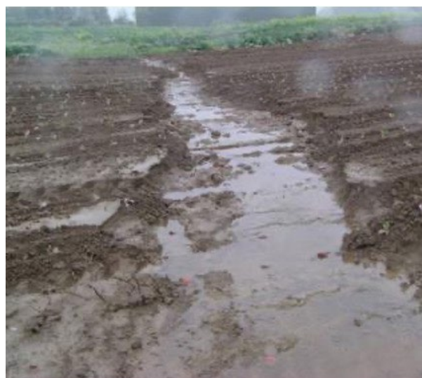
Figure 3.1: Damage caused by overland flow during a rain event flowing through a cropped block.
