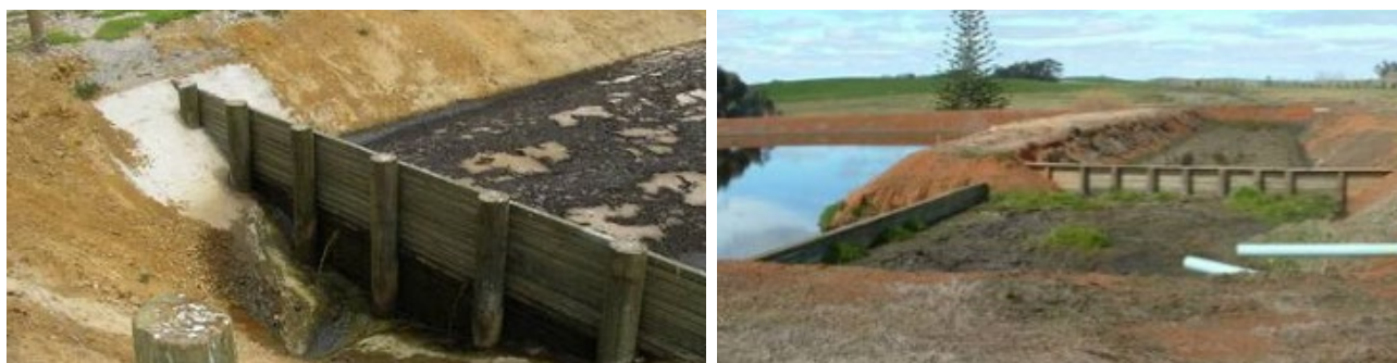
Figure 4.2: Weeping wall for dairy farm effluent, showing the wall, and sludge collected. Liquid seeps through the wall, to then be held ready for land application. Used with permission from Northland Regional Council.
