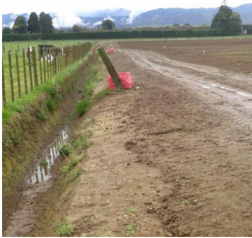
Figure 6. Cropping block before buffer strip installed. Photograph taken in November 2015.
