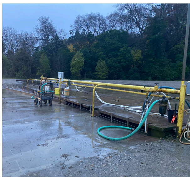
Figure 3.7: Washdown pad. Photo courtesy of Leaderbrand Gisborne.
