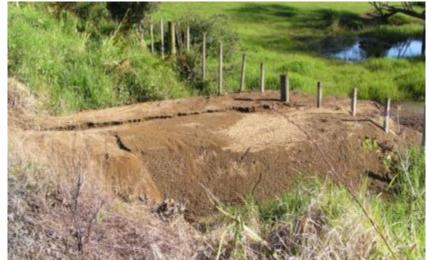
Remember – access ways are there to provide for vehicle crossings, they are not a discharge point for stormwater.
