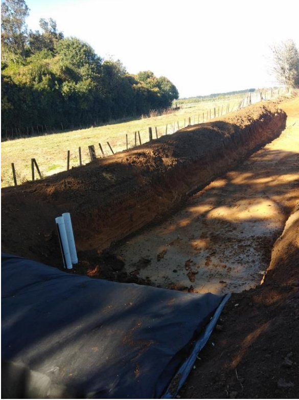
Image 3. Recently installed Sediment Retention Pond on Home Farm.
