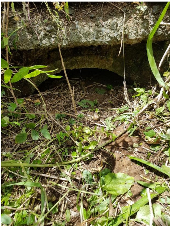
Image 2. An example of a blocked culvert on Home Farm.
