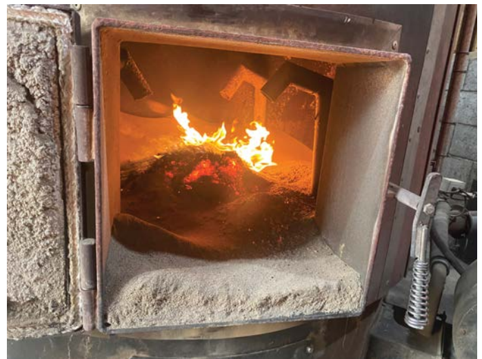
JS Ewers has converted its 30-year-old coal boilers to take wood pellets
