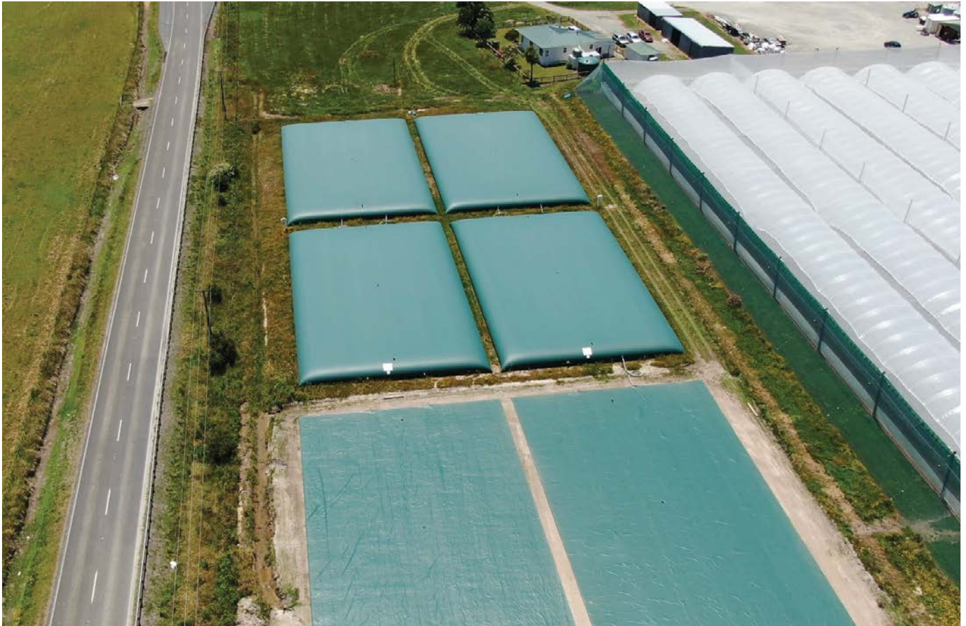
Flexi Tanks NZ's bladder storage is found throughout New Zealand, such as these (1 million litres each) at a Tolaga Bay covered crop operation. Flexi Tanks NZ's Anton Meier says the installation takes just hours to complete. The tanks, manufactured by France's Labaronne since 1959, have proven extremely tough and long-lasting. Photo by Flexi Tanks NZ
