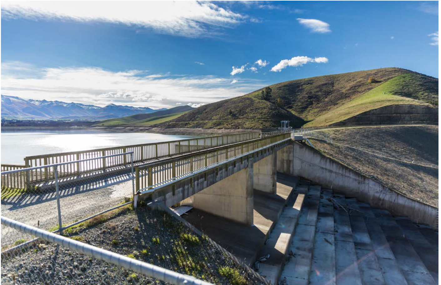
The Opuha Dam's 7-megawatt turbine generates power for the local network, on average powering 4000 to 5000 homes
