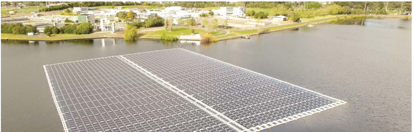
Believed to be the only floating solar array in operation in New Zealand, Watercare's Rosedale Wastewater Treatment Plant in Albany is a great example of using a pond's surface area to generate power for on-farm use and / or export to the grid, which can partly offset the lost production from the pond area. Photo courtesy of Watercare
