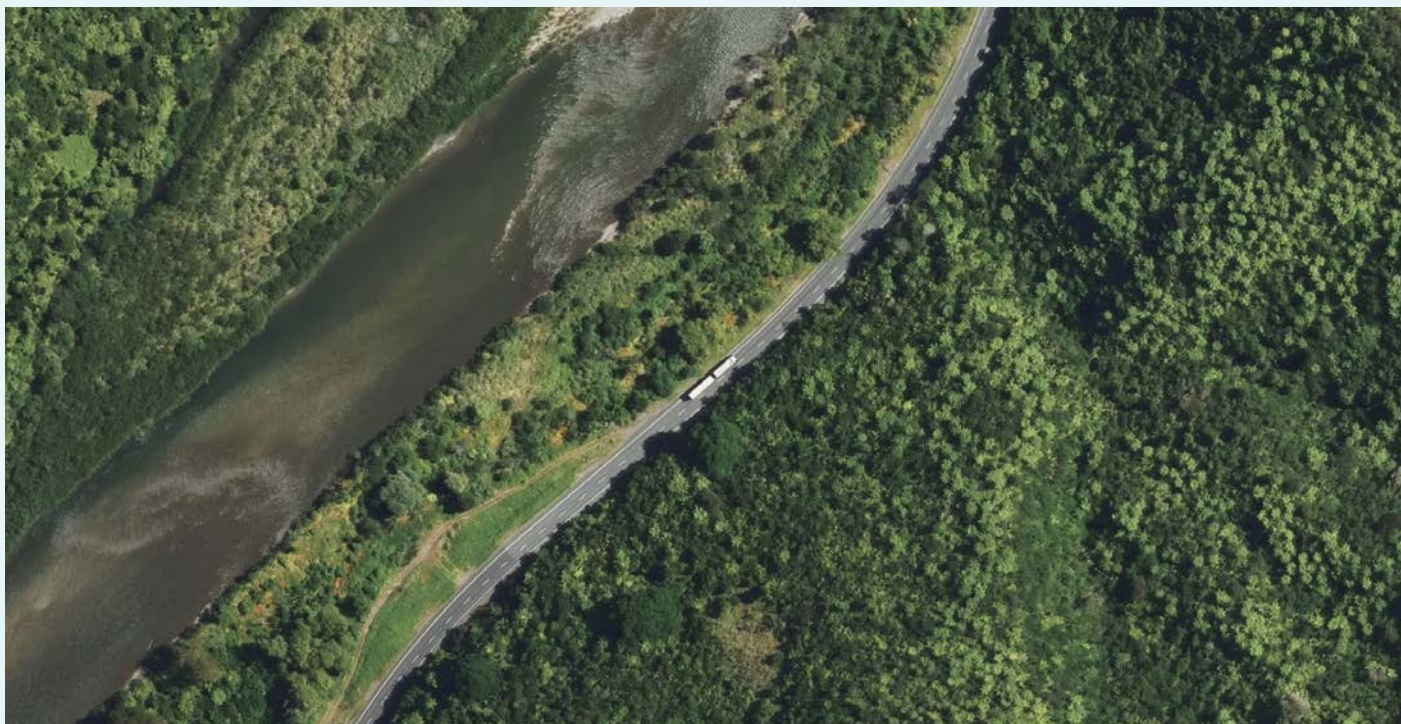
Slips along State Highway 2 next to the Waiōeka River can disrupt movements of perishable fresh produce. Photo courtesy of Toitū Te Whenua Land Information New Zealand
