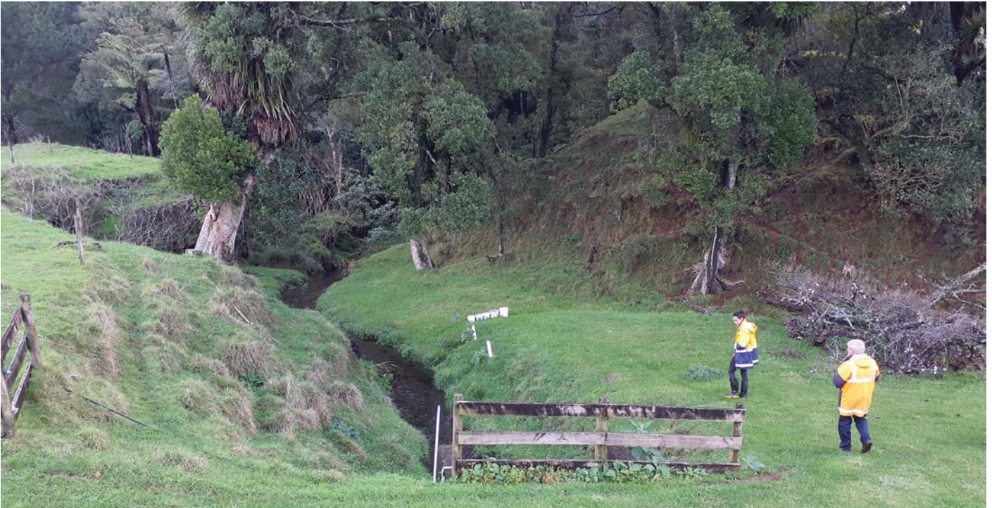
WSP inspectors assessing flood control
