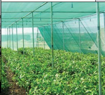
FLAT ROOF SHADE HOUSES
