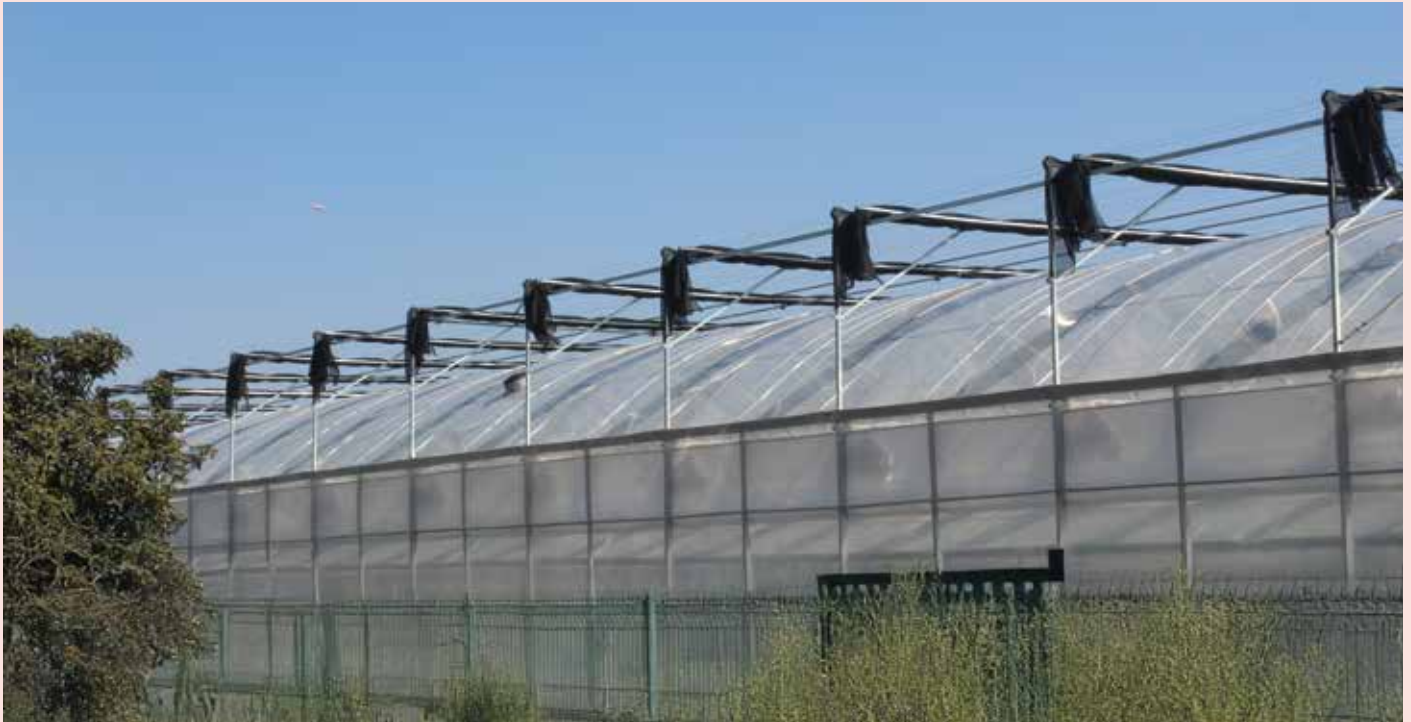
Support to shade netting over the greenhouse roof during a field visit near Yancheng
