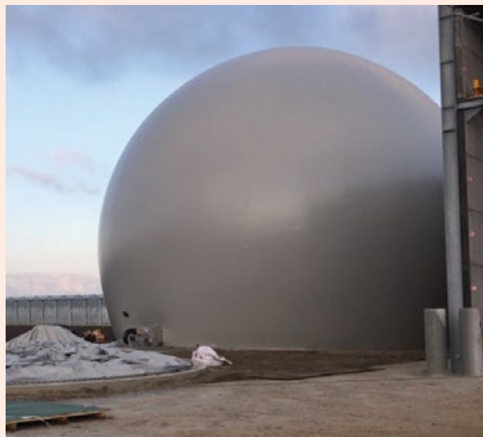
The spheres pictured here are balloons that store CO 2
