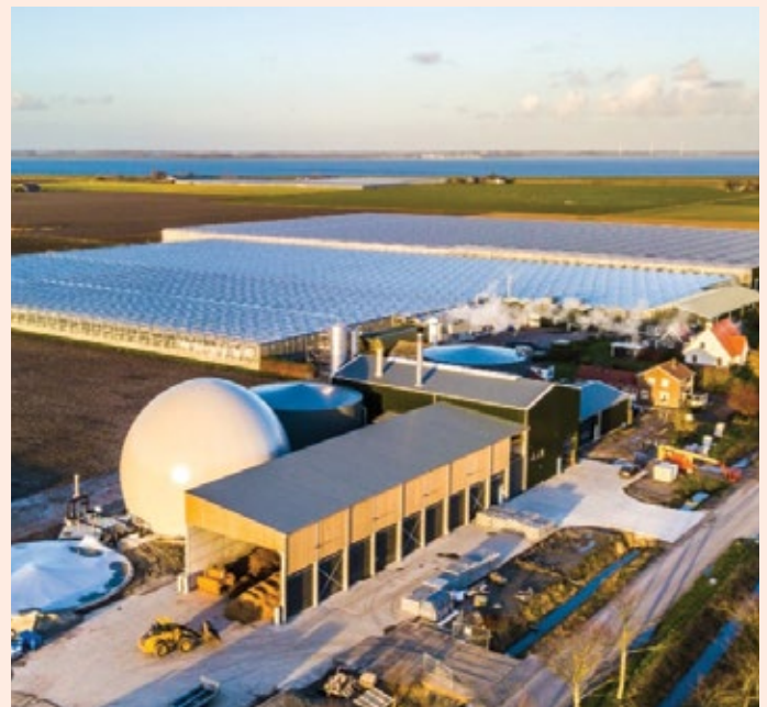
Dutch company DES's biomass installation for waste wood with a CO 2 capturing facility
