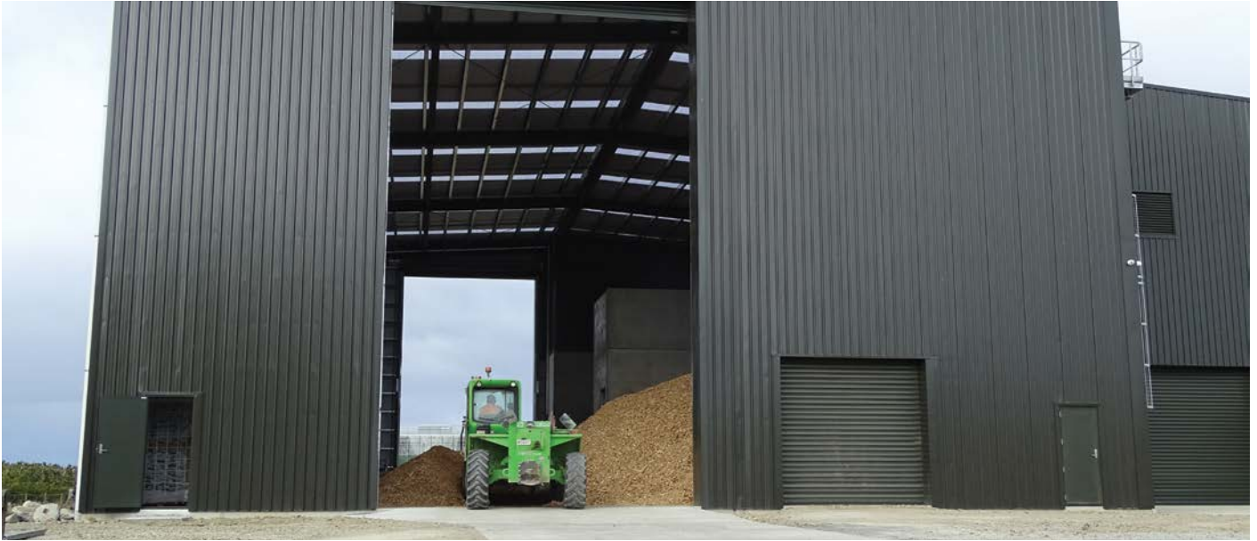
The new biomass facility at JS Ewers replaces coal with woodchip
