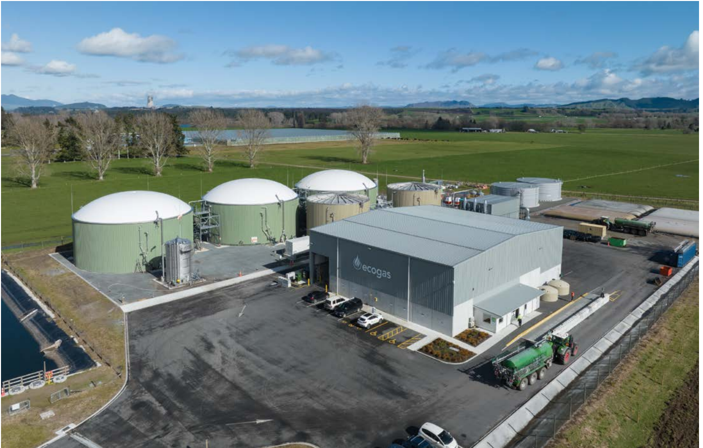
T&G's partnership with Ecogas will see its Reporoa greenhouses supplied with hot water, biogas and CO 2
