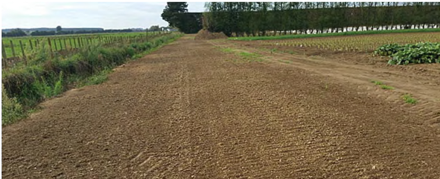
A well flattened and graded zone prior to seeding with grass. Land shaping in this manner will promote sheet flow of run-off over the entire buffer and minimise the formation of channels
