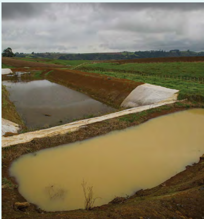
Sediment traps showing fine silt and coarse sediment collection areas
