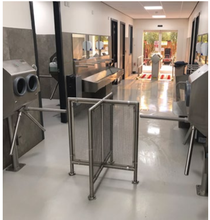
A UK greenhouse's hygiene street based on Royal Brinkman's HortiHygienz concept (forced soap handwash, final disinfection of hands and brush soles before continuing)
