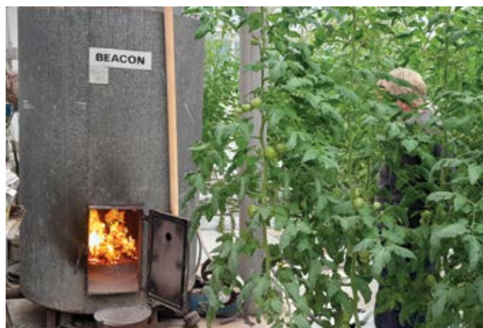
The re-purposed Beacon coal boiler now runs on wood pellets
