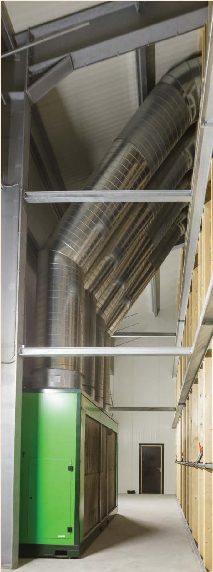
A Tolsma potato storage ventilation system. Photo courtesy of Tolsma Australia
