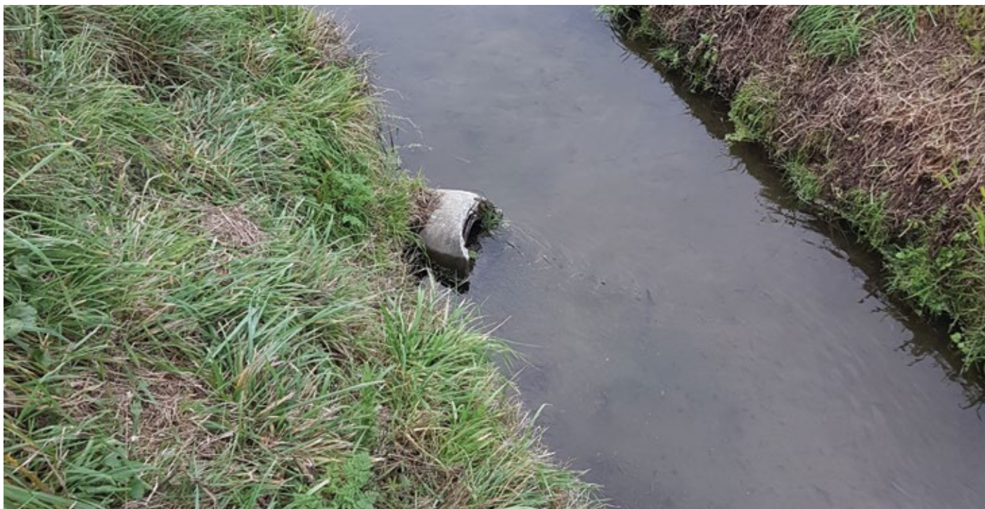
A tile drain exit point
