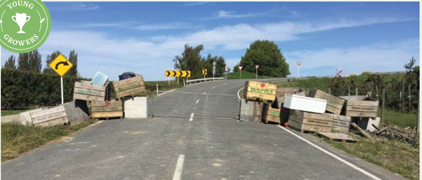
Damage to infrastructure such as the Brookfields bridge makes container deliveries to port or picking up bins and delivering them to the packhouse chaotic
