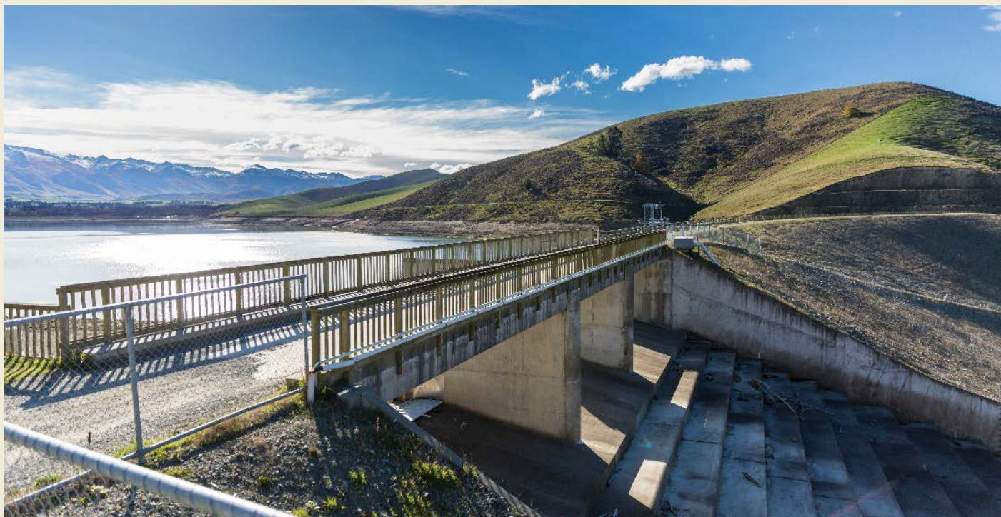
The Opuha Dam's 7-megawatt turbine generates power for the local network, on average powering 4000 to 5000 homes
