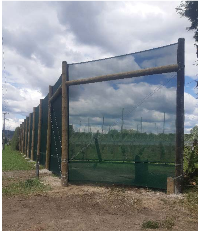
A recently constructed artificial shelter near a roadside. Photo courtesy of BK Developments
