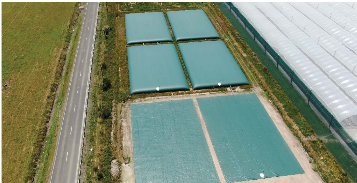
Flexi Tanks NZ's bladder storage is found throughout New Zealand, such as these (1 million litres each) at a Tolaga Bay covered crop operation. Flexi Tanks NZ's Anton Meier says the installation takes just hours to complete. The tanks, manufactured by France's Labaronne since 1959, have proven extremely tough and long-lasting. Photo by Flexi Tanks NZ
