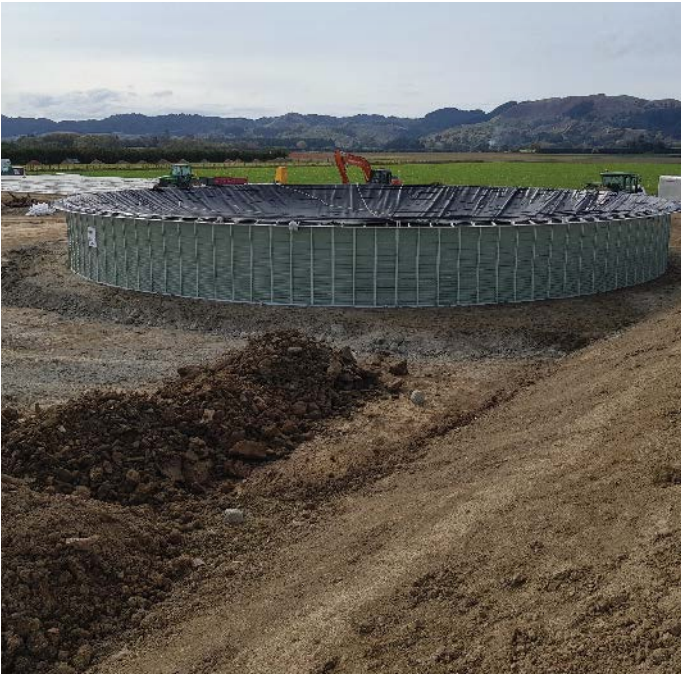
A large KlipTank installation in New Zealand. Photo courtesy of KlipTank
