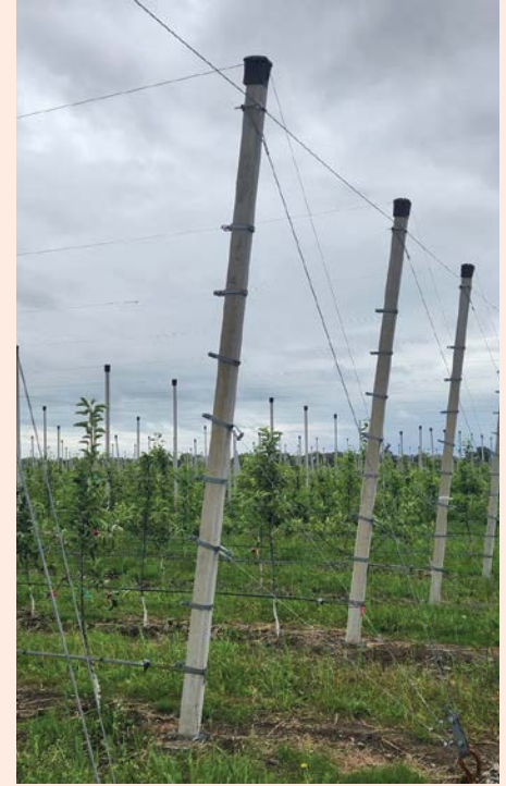
Concrete posts have become available in New Zealand, creating a long-lasting and environmentally friendly alternative
