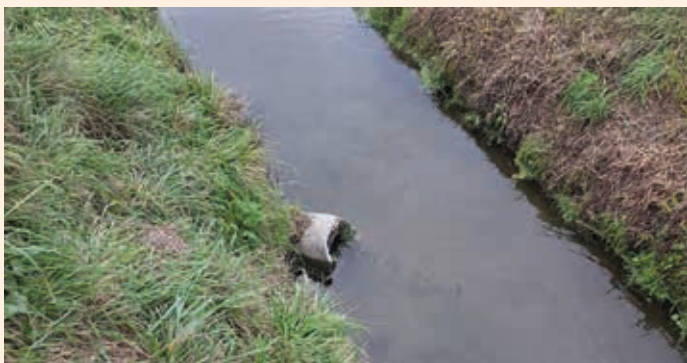
Figure 2 A subsurface drainage line exiting a farm property into a waterway
