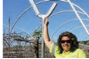
Hooks built into the tunnel house structure will support the catchment to funnel water into the nearby reservoir
