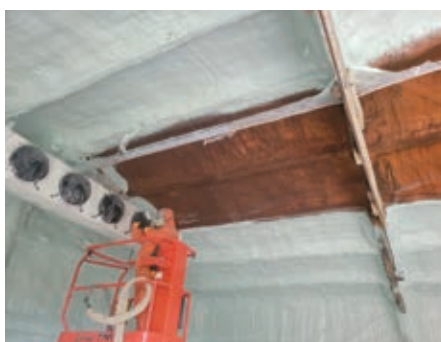
Fresh spray foam being applied
