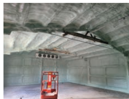
Finished Fruit Storage shed!
