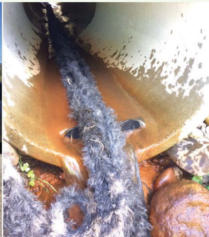
A fish ladder in place in a culvert to enable the tiny fish to 'climb' or swim through the culvert, upstream to breed
