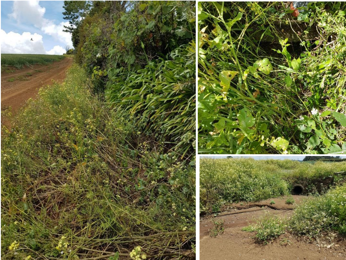
Figure 3. From top left clockwise: i) Overgrown and shallow interception drain along southern boundary. ii) Blocked culvert from southern boundary interception drain. iii) Culvert leading to SRP 2.
